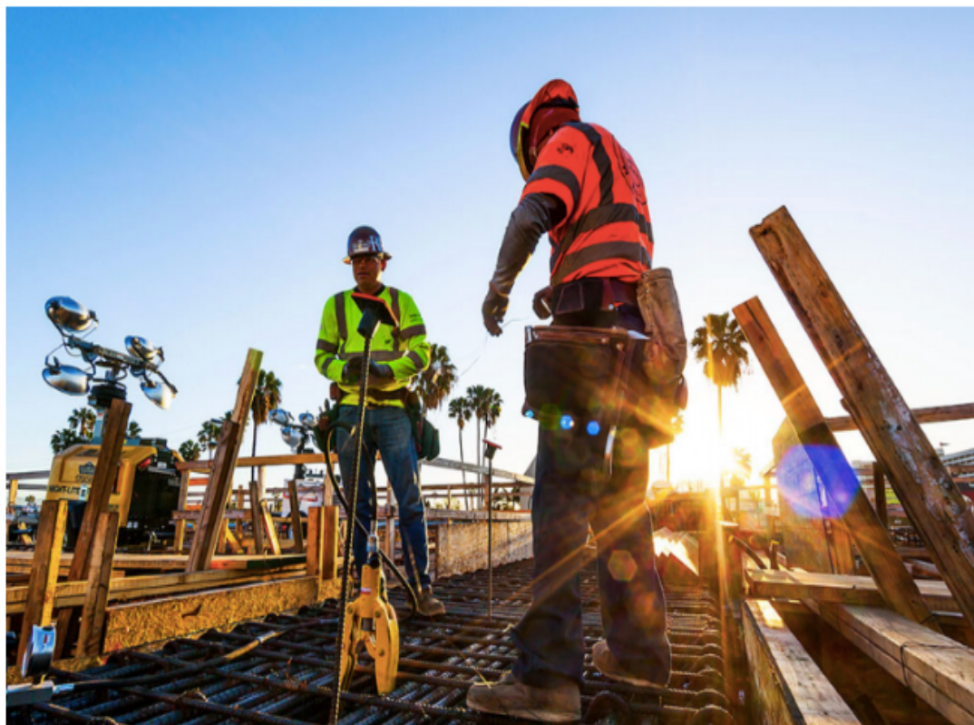
Construction along Crenshaw/LAX Transit Corridor. Image: HNTB
